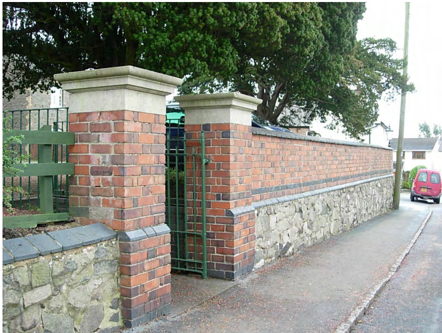
This solid brick wall that stand on a granite base is a dominant feature fronting the former village primary school and should be retained.
