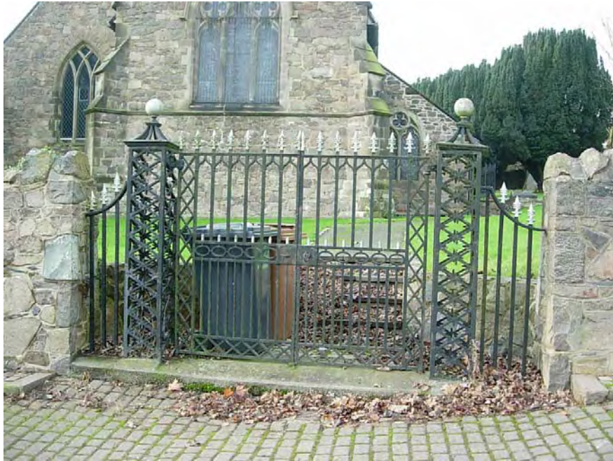
Cast iron gates circa 1820 with their pierced openwork side piers. The Grade 2 listed gates are an excellent feature sited on the east side of St Michael's Church.
