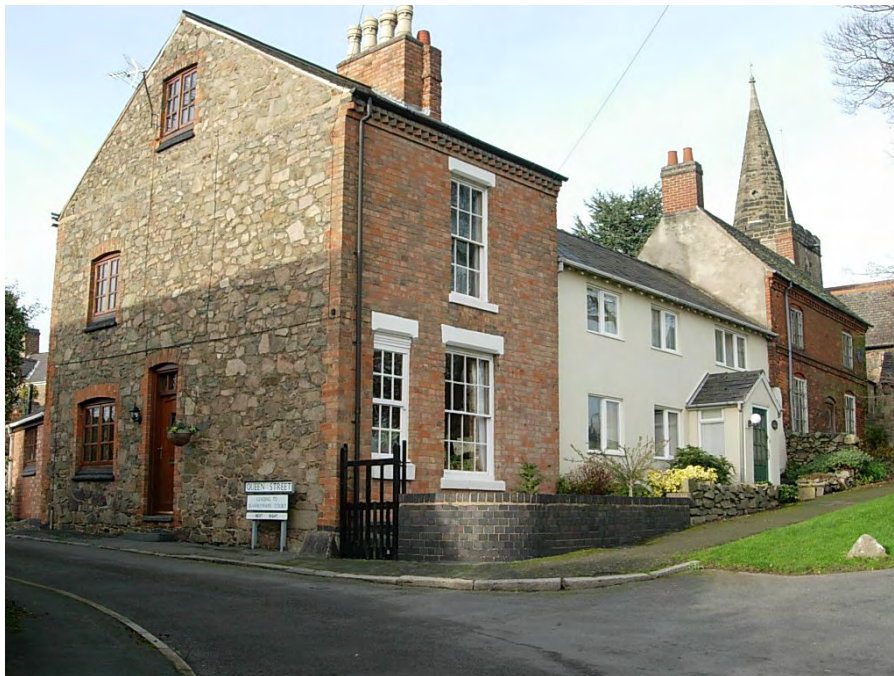
The dwellings adjacent to the church lichgate provide a fine setting for the church with their different roof heights and materials.
