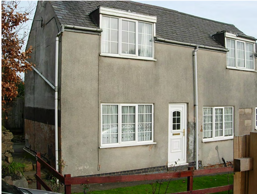
52 The Green that was originally two cottages that has lost its traditional character with its conversion into a single property and use of modern materials.
