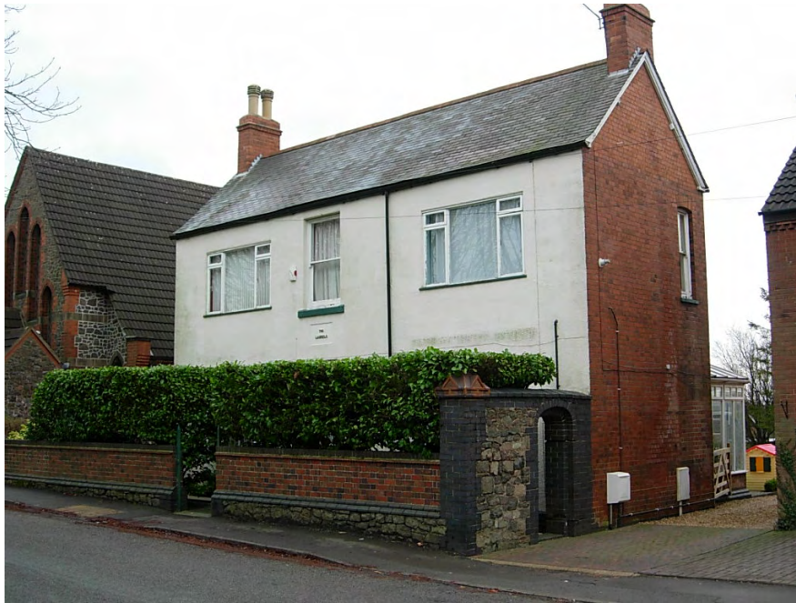
The Laurels, 40 Main Street is a fine building although it has lost some of its traditional character with the insertion of two large windows on the front elevation.
