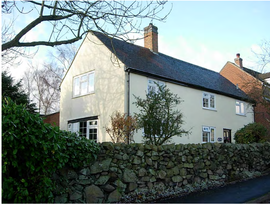
29 The Green suffers from overly large window openings in the gable and plastic windows.
