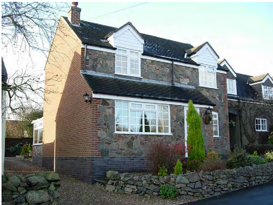
31 The Green has many non traditional features that detract from the conservation area. They include half dormers, overly large window openings and inappropriate modern materials.
