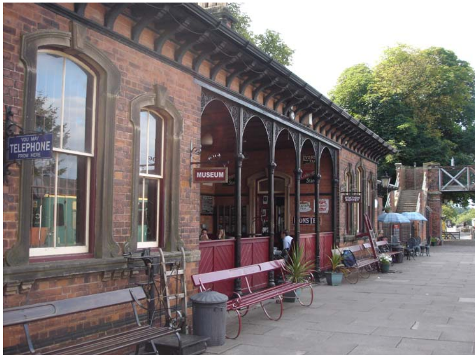
The platform side of Shackerstone Station showing a 5 bay open centre with cast iron columns.
