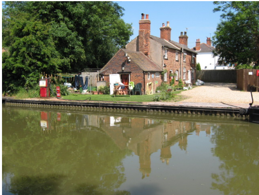
The setting of original canal side buildings at Stoke Golding has been spoilt by sheet piling running along the edge of the canal.
