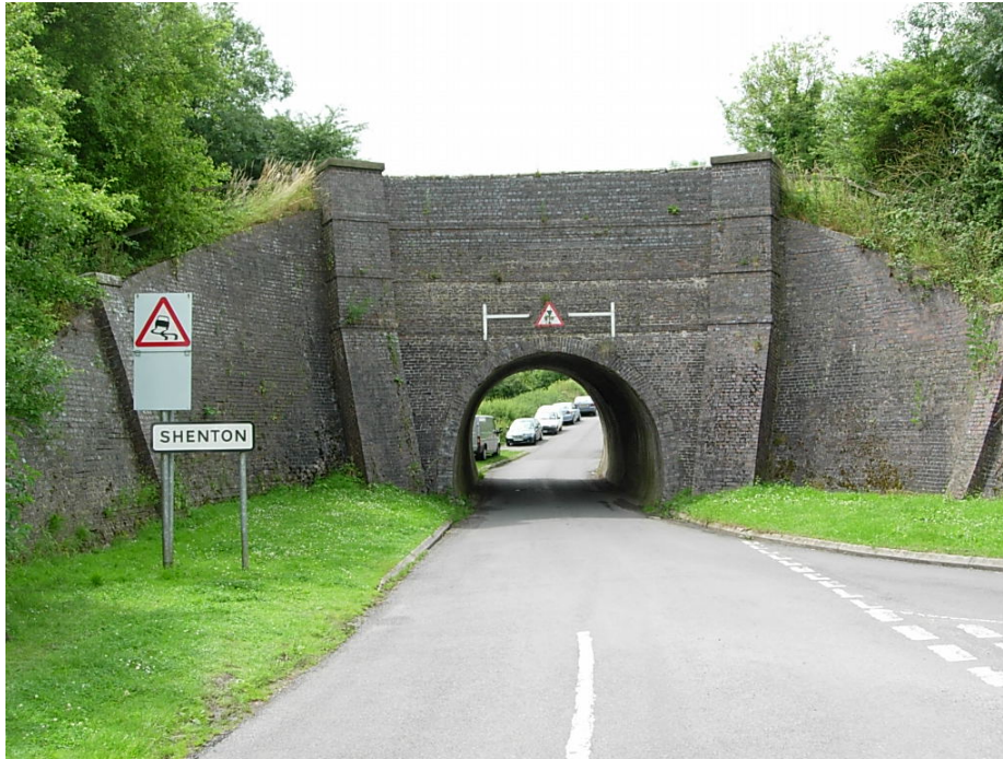
One of two aqueducts on the Ashby Canal sited at Shenton and Shackerstone. This one built in brindle blue brick on a high embankment which reaches a height of 20 feet or more spans the road into Shenton.
