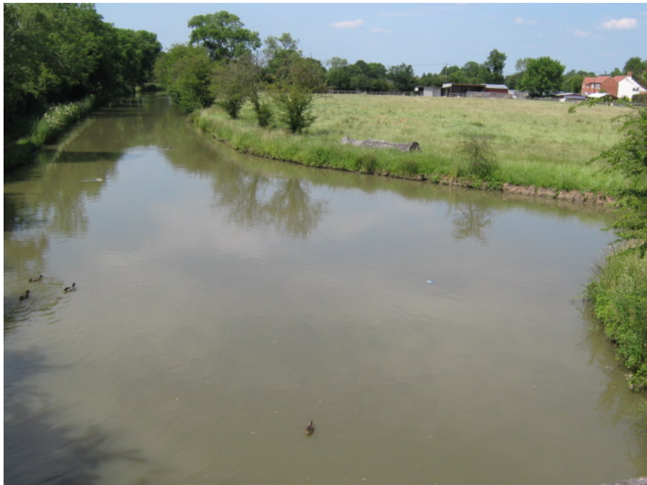
One of several winding holes on the canal that allows barges to turn around.
