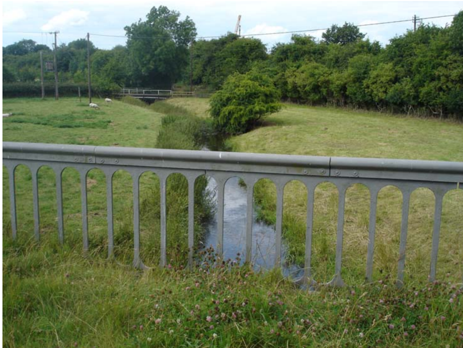
The cast iron railings are a fine heritage feature that were saved and renovated under the Borough Council's Environmental Improvement Programme.
