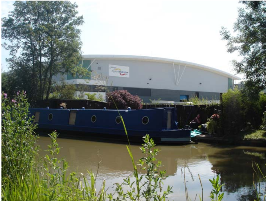
Modern warehouses abutting the canal generally have a detrimental impact on its rural character.
