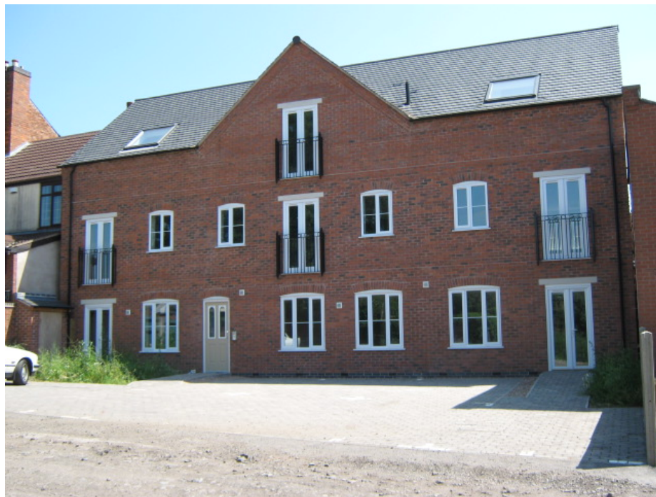
A recent building added to the Hinckley Wharf complex which does not reinforce canal side architecture.
