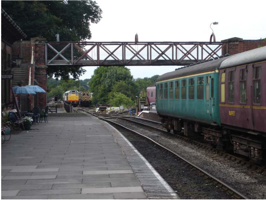
Shackerstone Station footbridge
