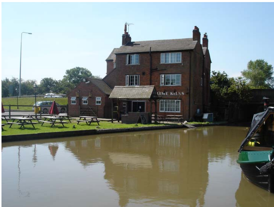
The three storey Lime Kilns Public House fronting Watling Street. The property presents a traditional appearance which is important to retain.
