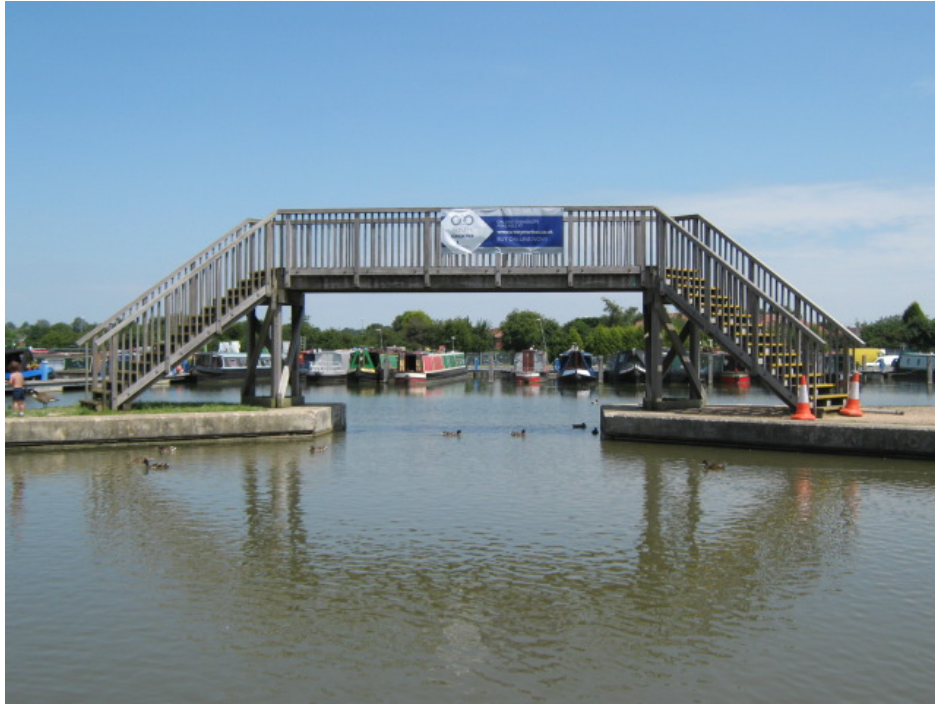
This timber bridge marks the entrance to the Coventry Road Marina.
