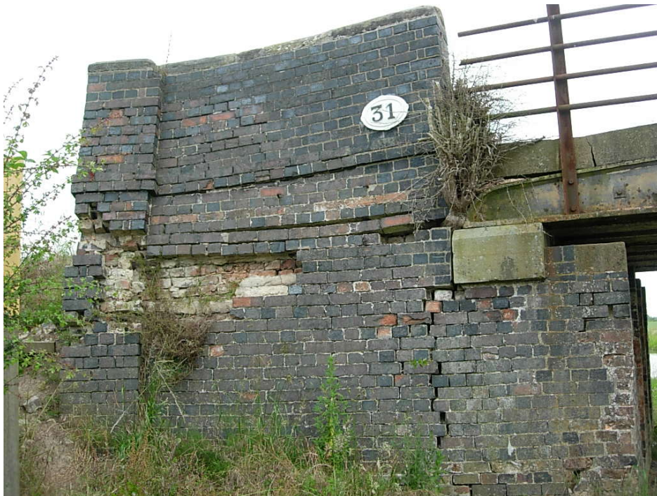
British Waterways has agreed to re-build the parapet and affected buttress in April 2010
