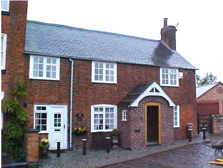
35 Chapel Hill has suffered from the installation of a modern door and construction of an over dominant front porch.
