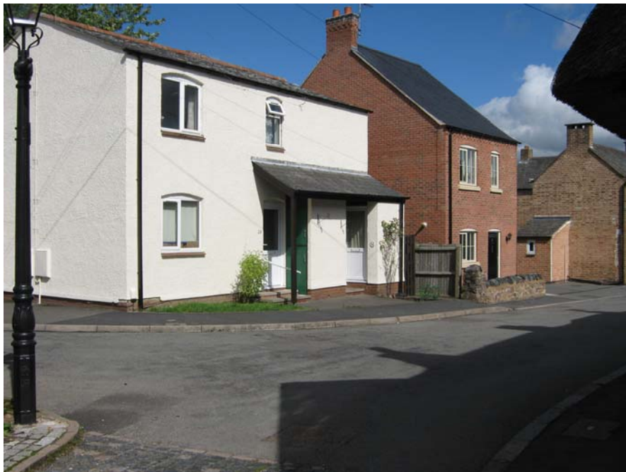
28 Chapel Hill is a modern white rendered dwelling which unfortunately has plastic windows, a front canopy and a shallow roof pitch.
