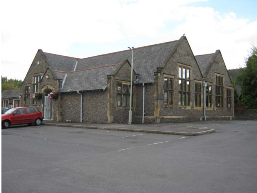
The former village school built in stone with ashlar dressings and slate roof is now used as Groby's village hall and parish council offices.
