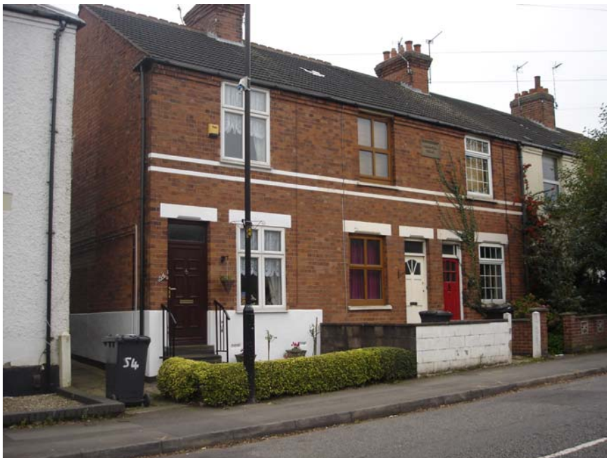
The unity of Victoria Stone Terrace has been lost due to modern improvements. The terrace, however, has retained its impressive chimney stacks.
