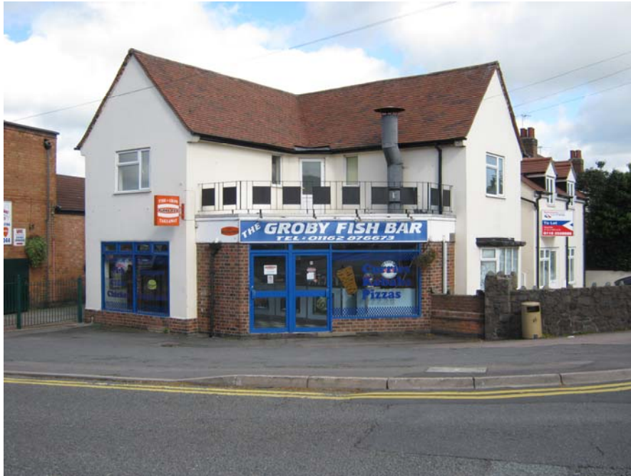
This inappropriate shop front added to 1 Newtown Linford Lane has a detrimental impact on the street scene by way of the over dominant signage, colour scheme, balcony and extractor flue.
