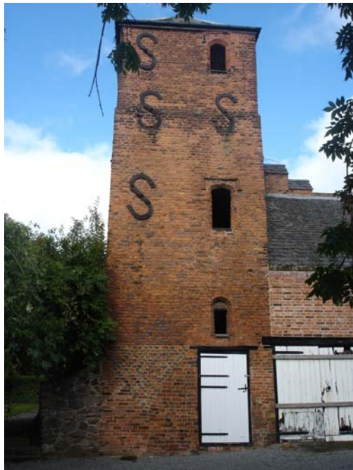
The imposing four storey Tudor tower abutting Groby Old Hall with its hipped roof is a landmark feature on Markfield Road.
