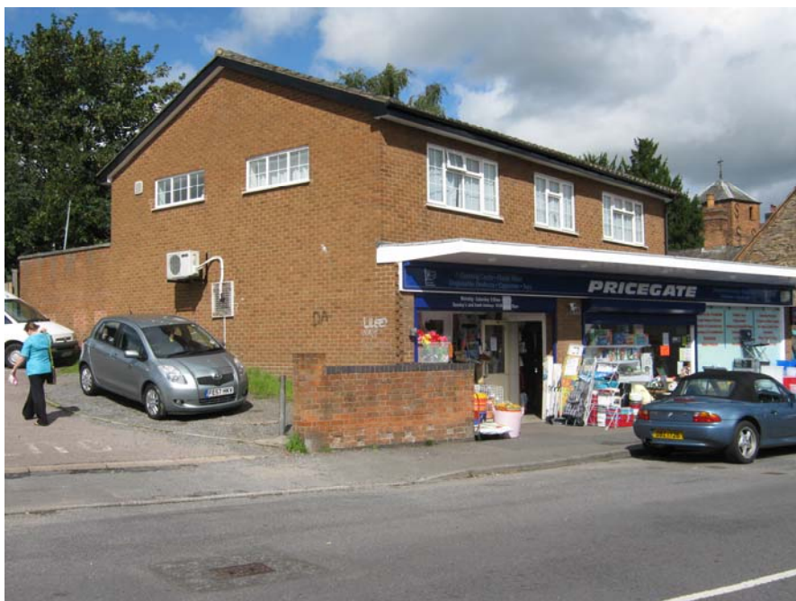
This large modern property and the external treatment of the shop front are far too brash and prominent in the centre of the conservation area. Consideration needs to be given to reduce its visual impact in the street scene.
