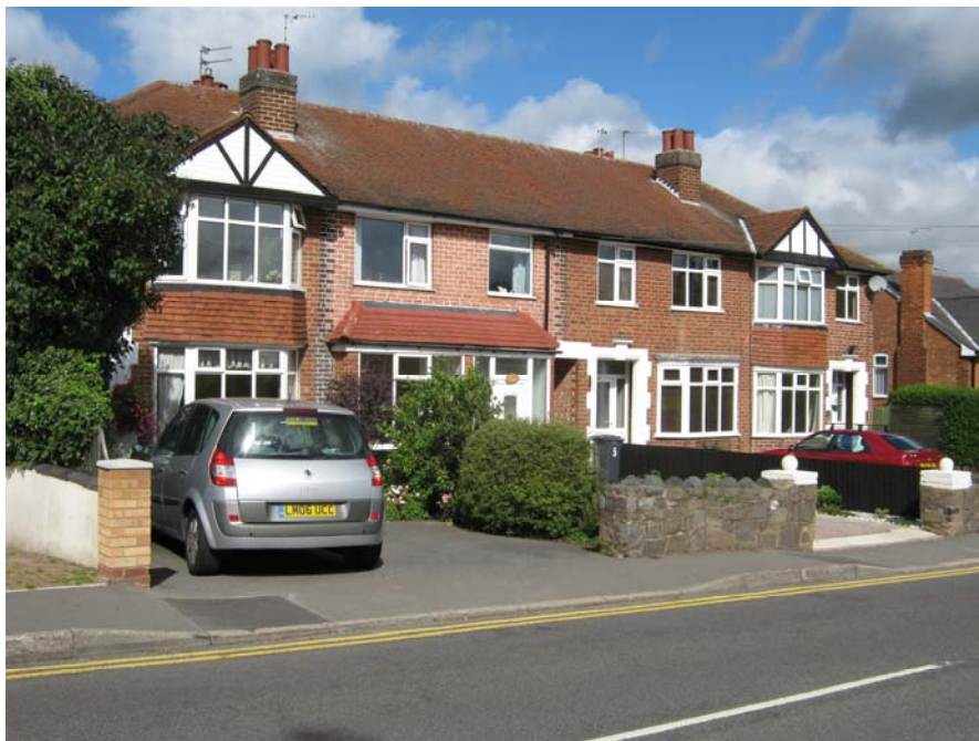
The unity of the terrace 3 – 9 Newtown Linford Lane has been lost due to modern improvements.
