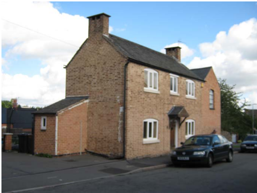
20 Chapel Hill is an early C19 Grade II listed building with a slate roof and two brick stacks. The gable fronting the carriageway has some fine cast iron glazing bar windows. Unfortunately, the property has lost its chimney pots.
