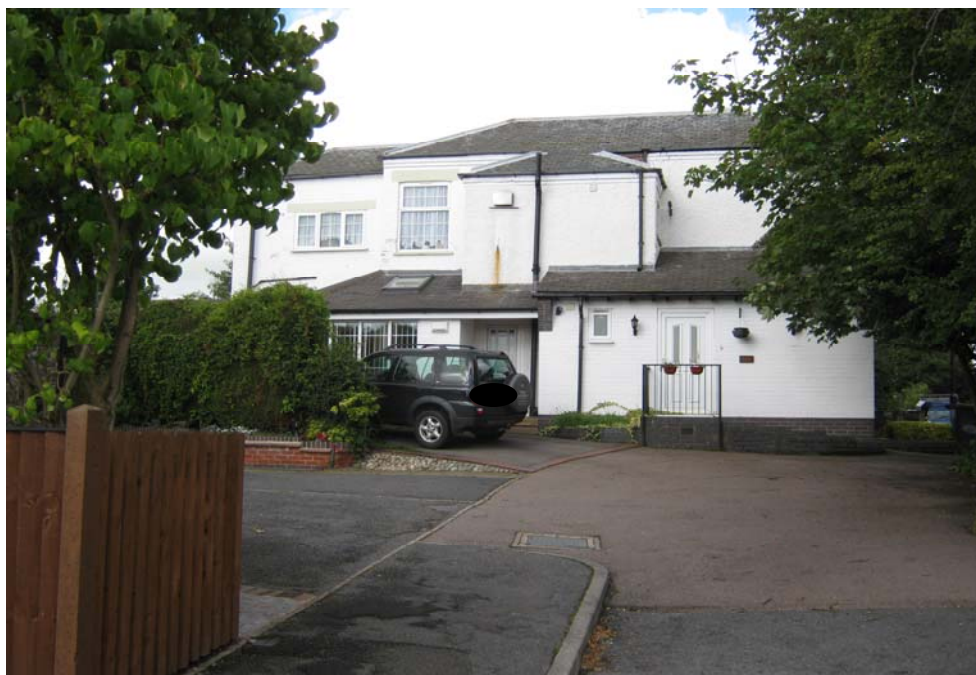
The large rendered property, 56 Leicester Road, has now been converted into two flats.
