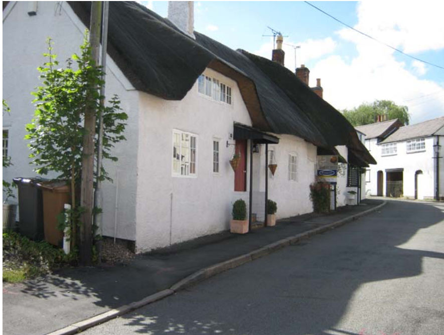
23 – 27 Chapel Hill are three C17 Grade II listed picturesque properties, originally timber framed, under-built in brick and rendered. The thatched cottages have eyebrow dormers both to the front and rear. Two of the front porches have thatched roofs and one, slate.
