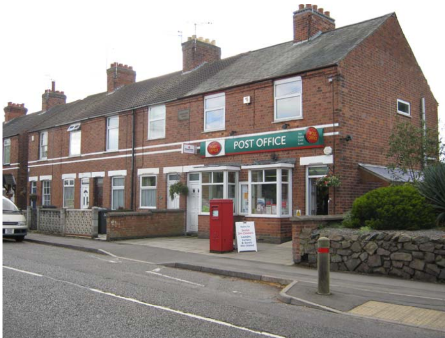
The bay window and over dominant shop fascia sign fronting the post office have a detrimental visual impact on the character of Victoria Terrace.
