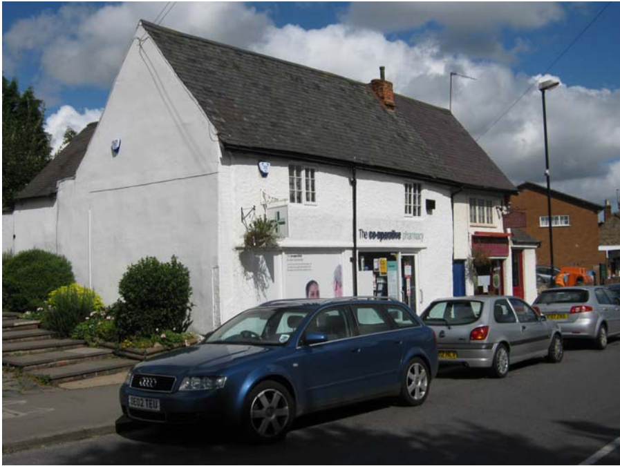
18 & 18a Ratby Road is a vernacular building that has been rendered and painted.
