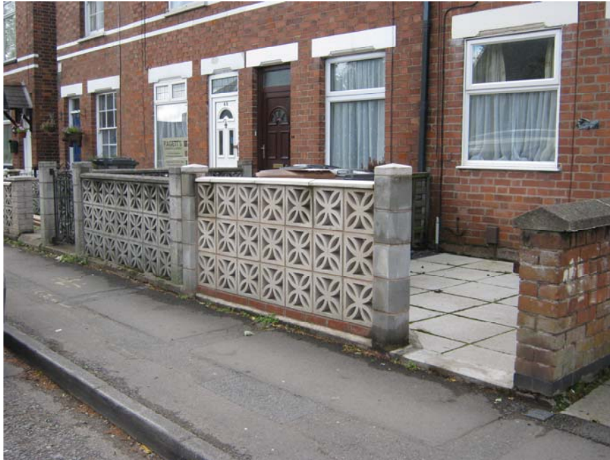
This particular wall treatment on Leicester Road is unacceptable clashing with the character of traditional stone walls in the conservation area.
