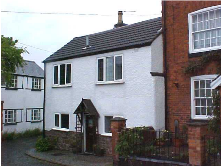
31 Chapel Hill was once a Grade II listed property built in red brick with slate roof with a south side façade jettied out with rough cast 1 st floor. However, the dwelling was de-listed due to its modernisation with concrete roof tiles and plastic windows.
