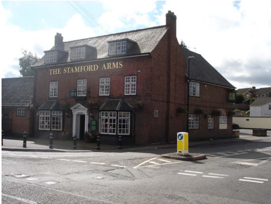
The Grade II listed late C18 Earl Stamford Arms Pub is built in red brick. It has a slate roof and 2 brick gable stacks. The roof was raised in C20 and 3 flat roof casement dormers were added.
