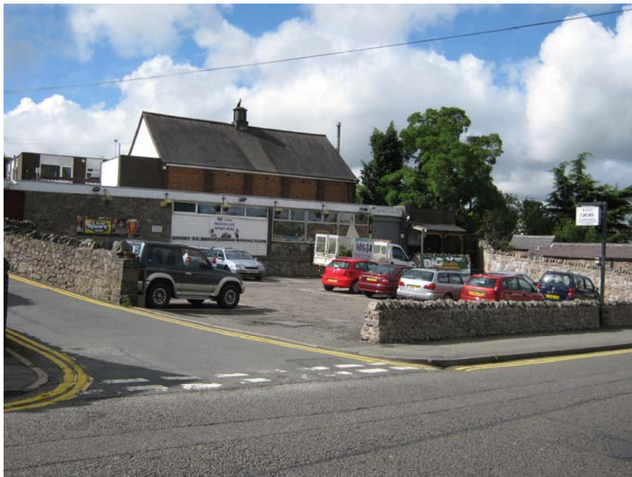
The flat roof front extension to the Ex-Sevicemens' Club sited opposite Newtown Linford Lane has an unfortunate detrimental effect on this part of the conservation area. The traditional stone walls, however, help delineate the Club's car park boundary.
