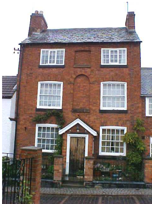
35 Chapel Hill is a circa 1800 Grade II listed house. The three storey property is built in red brick, slate roof and has two gable stacks. The central planked door has been fitted into a late C19 gabled porch with terracotta lintels.
