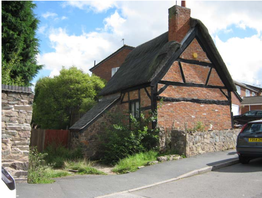
The Grade II listed Blacksmith's Cottage on Rookery Lane. The late C17 timber framed property with brick noggin and thatched roof has a single gable stack. This attractive little thatched cottage, that was once the site of the village blacksmith, was restored around 1980.
