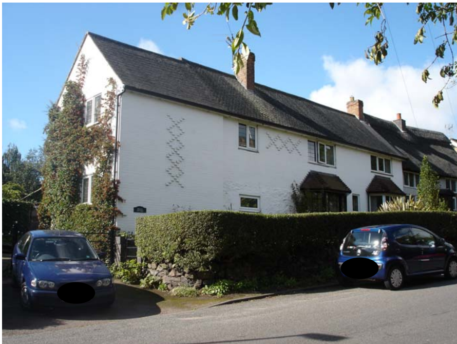
13 Markfield Road is a large imposing dwelling with two front bay windows and a fine privet hedge. The property is rendered, painted white with a slate roof and interesting diaper brickwork.
