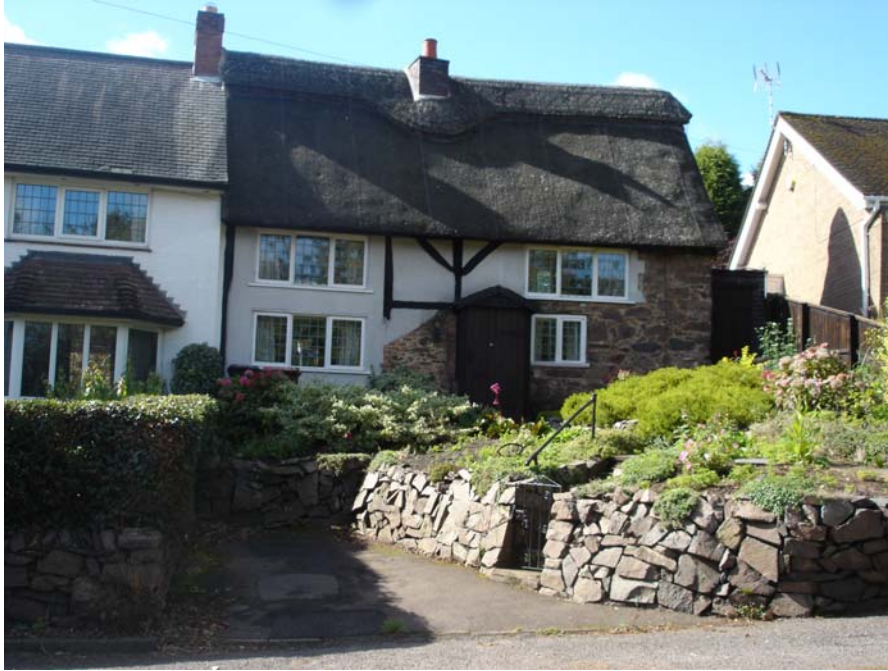
This charming thatched cottage, 15 Markfield Road, has one half of its front elevation built in stone and the other rendered.
