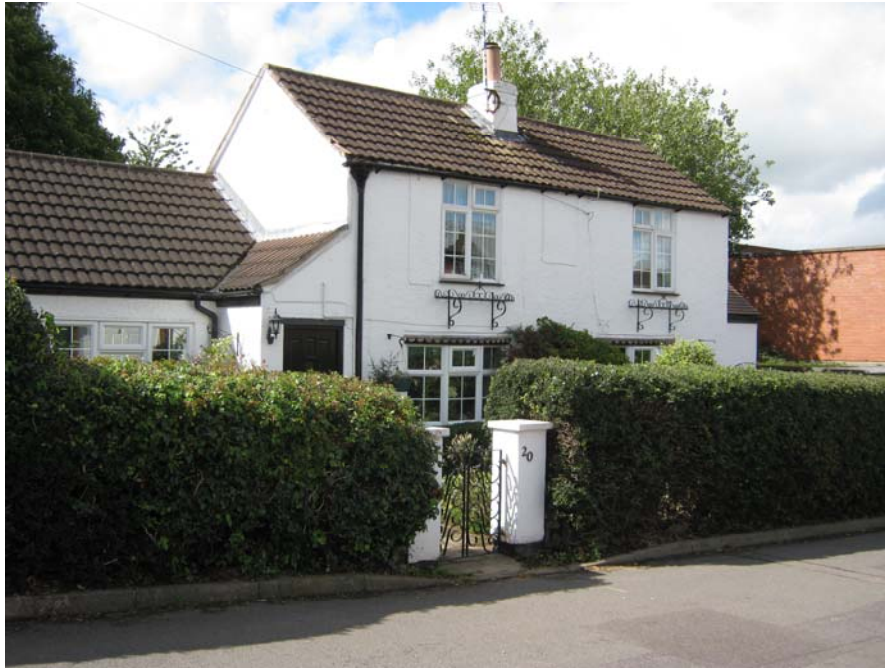
This cottage on Rookery Lane has lost its traditional character with the use of concrete roof tiles and installation of bow windows.
