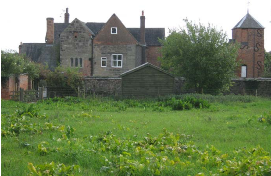
North-west view of Groby Old Hall and tower showing the right hand gable has been raised with brickwork.
