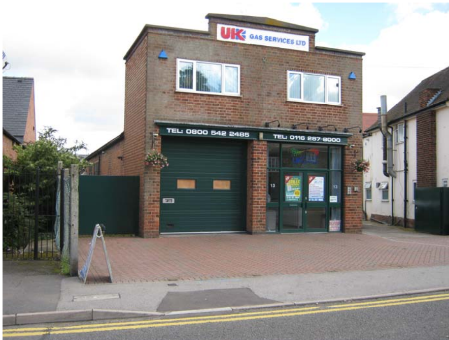
The commercial premises on Leicester Road is a particularly unattractive property in the conservation area due to its modern design, siting and poor surface treatment.
