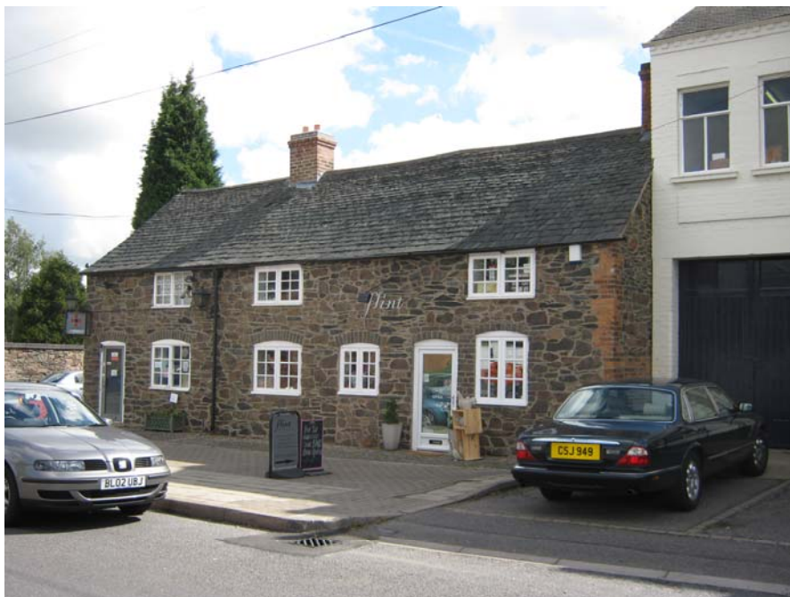
The cottages, 11 & 15 Ratby Road, are simplistic in their design and choice of natural materials although the street doors are out of character.
