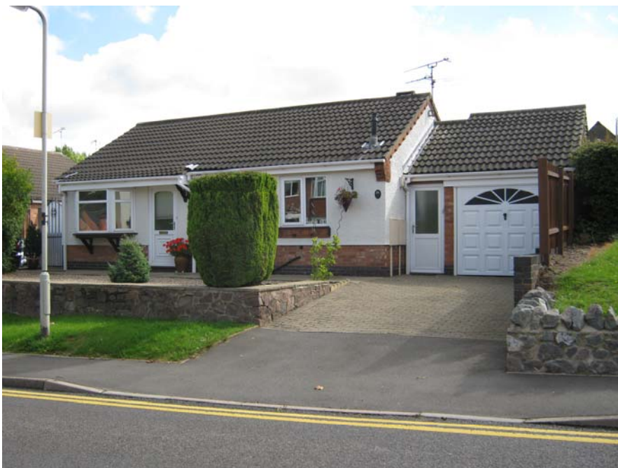
2 Newtown Linford Lane and the adjacent modern housing development do not reflect the character of the conservation area.
