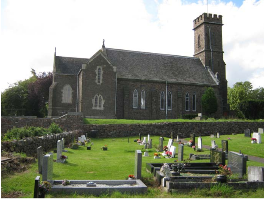
The Grade II listed parish church of St Philip & James built in 1840 in random coursed Mountsorrel granite with sandstone ashlar dressings and Swithland slate roofs. The tower has an embattled parapet which is visible from a number of vantage points throughout the settlement.
