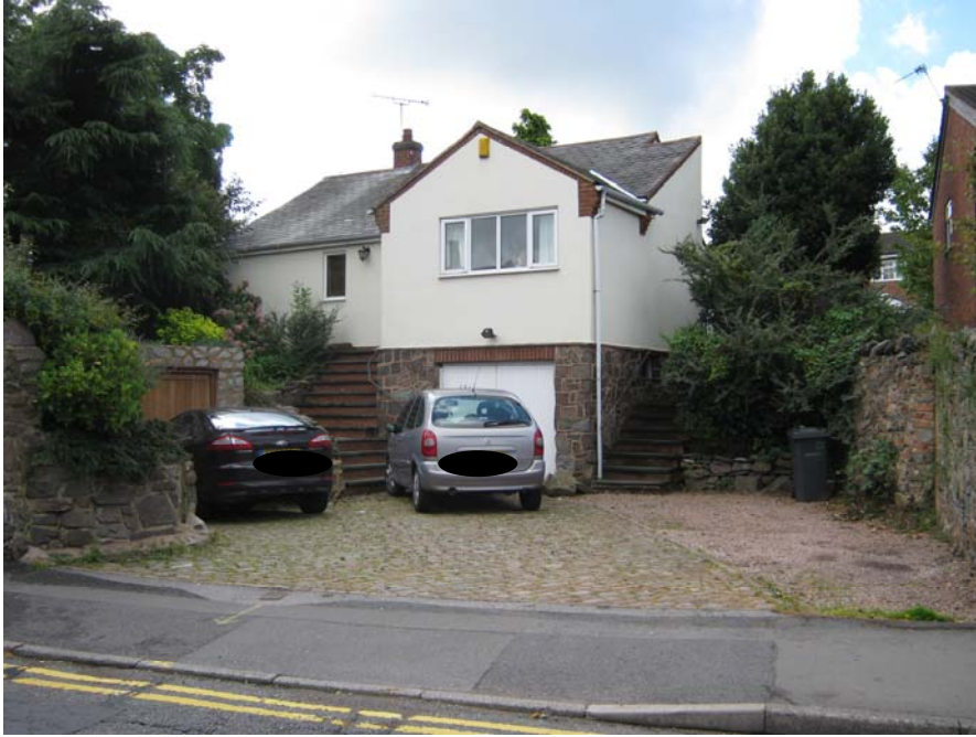
The half rendered split level bungalow, 12a Leicester Road, with its integral garage does not reflect the traditional character of the conservation area.
