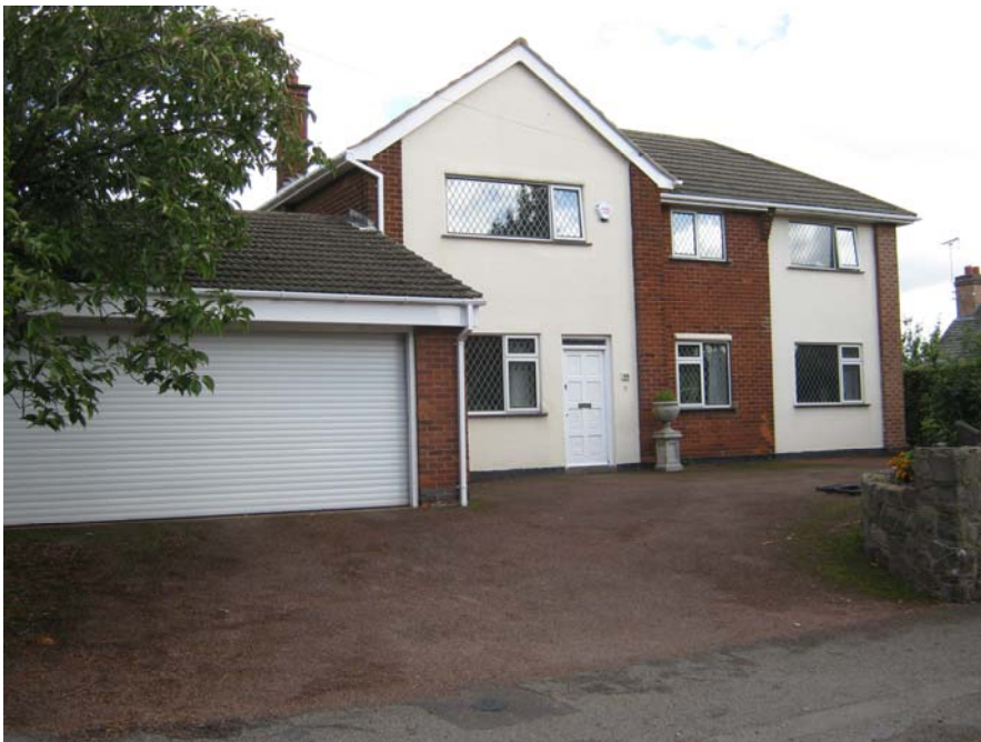
55 Leicester Road is a large detached modern dwelling that would have been better sited outside the conservation area due to its design and choice of materials.
