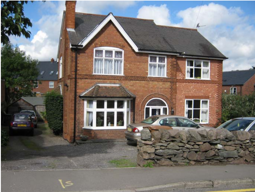
11 Newtown Linford Lane is a classic detached dwelling built in the early 20 th century that has had a recent side extension added.
