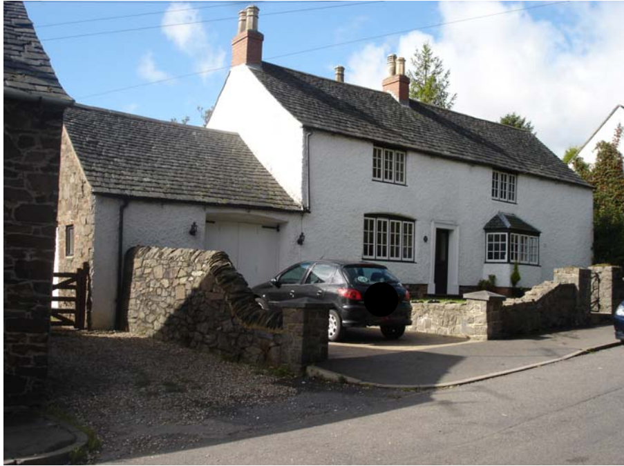
11 Markfield Road is a large rendered dwelling, painted white, with a stone plinth, slate roof and stone boundary walls. The property still has chimney stacks and pots and a front bay window has been added.
