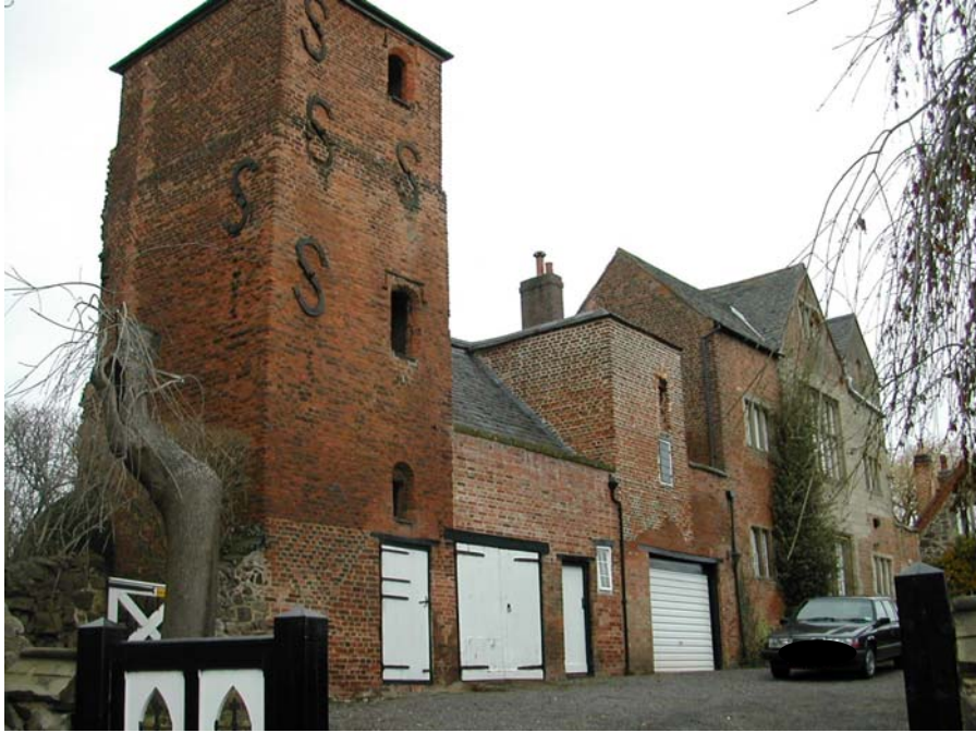
The Grade II* listed Groby Old Hall is a late C15 manor house built with red brick in English bond with some diaper work in black brick. The dwelling was originally the home of the Grey family with associations with the nine day queen, Lady Jane Grey. The Manor courts were formerly held in the room called the Old Hall. The property was altered C17, restored 1858 with some later C20 alterations.
