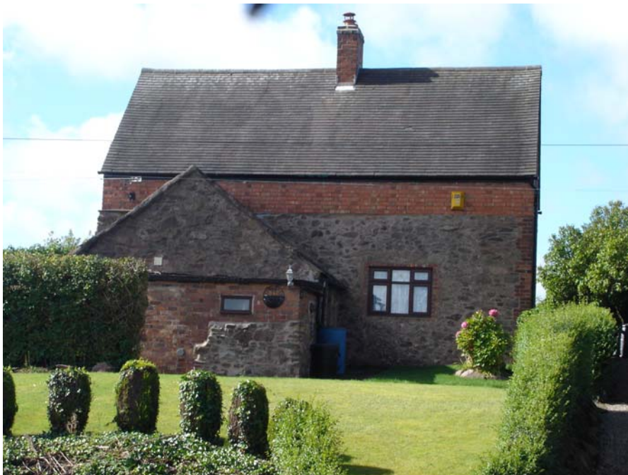
The stone property, 33 Markfield Road, showing its roof has been raised in brick and re-roofed with clay tiles.
