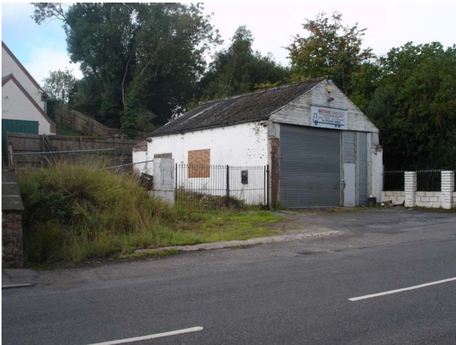
This former motor vehicle repair garage on Markfield Road is a particularly unattractive building in the conservation area. The site has potential for redevelopment.
