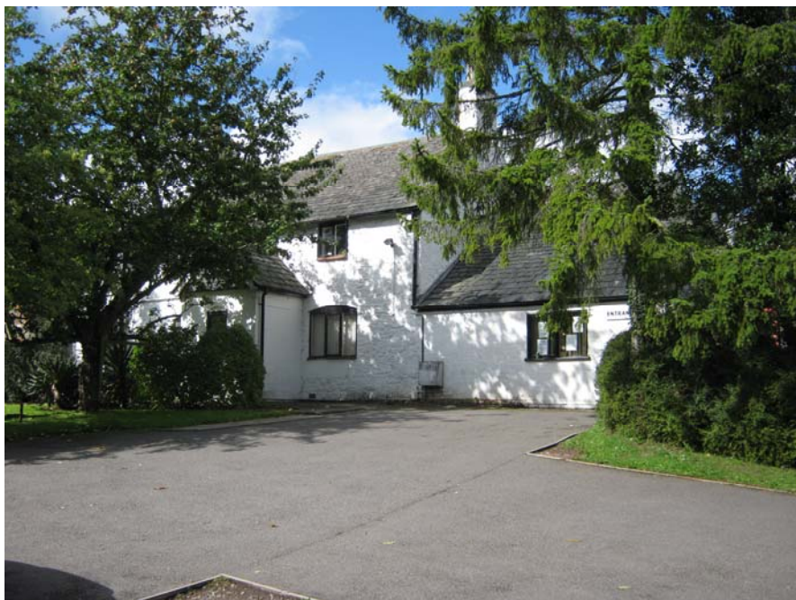
26 Rookery Lane is a late C18 Grade II property that has rubble stone walling with brick dressings, a Swithland slate roof and two brick painted gable stacks. The building is now a doctors' surgery.
