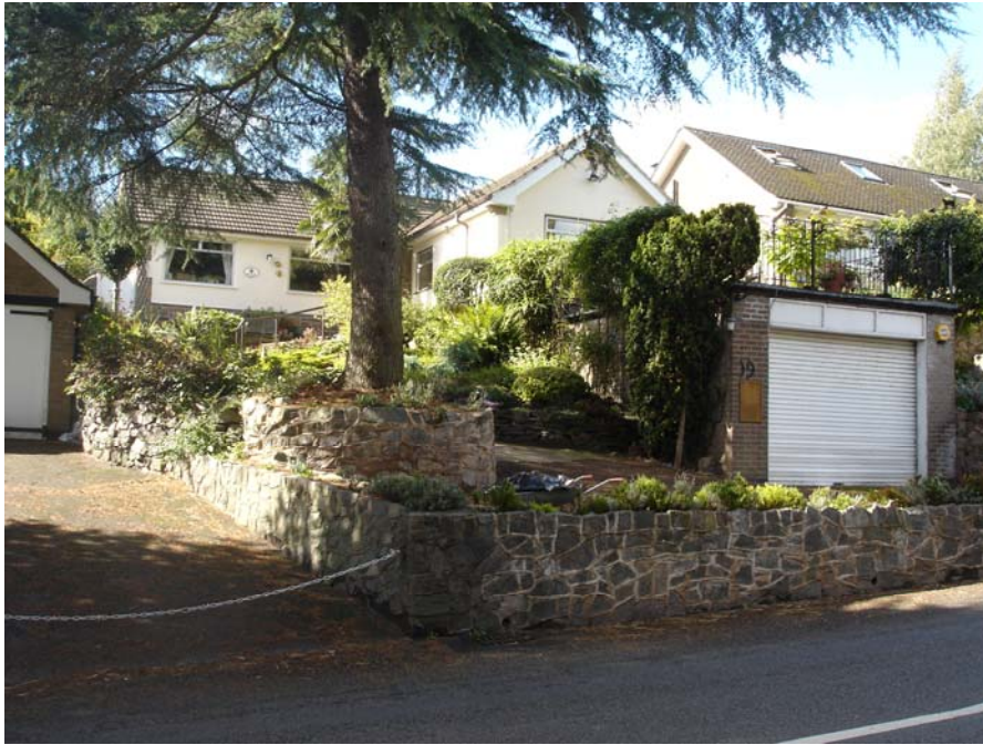
The brick garage fronting 19 Markfield Road does not respect traditional character of the conservation area in its form or siting.
