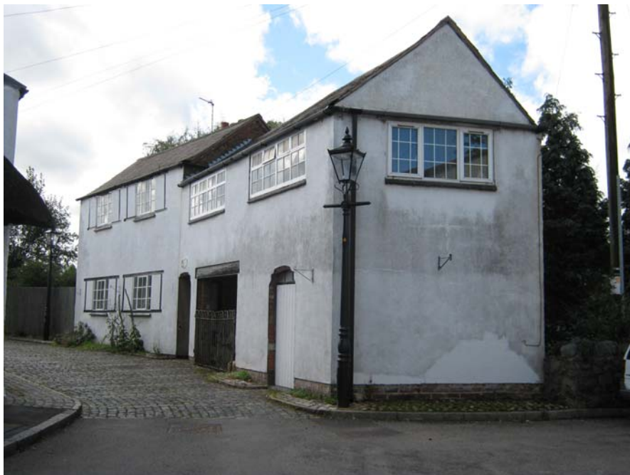
30 Chapel Hill was once a framework knitter's cottage. This is evident from its large rectangular window openings, several of which have now been reduced in size.
