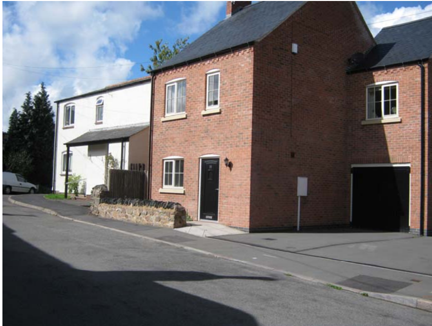
24 Chapel Hill is a modern house built with natural materials, unfortunately, the integral garage is not a traditional feature in the conservation area.
