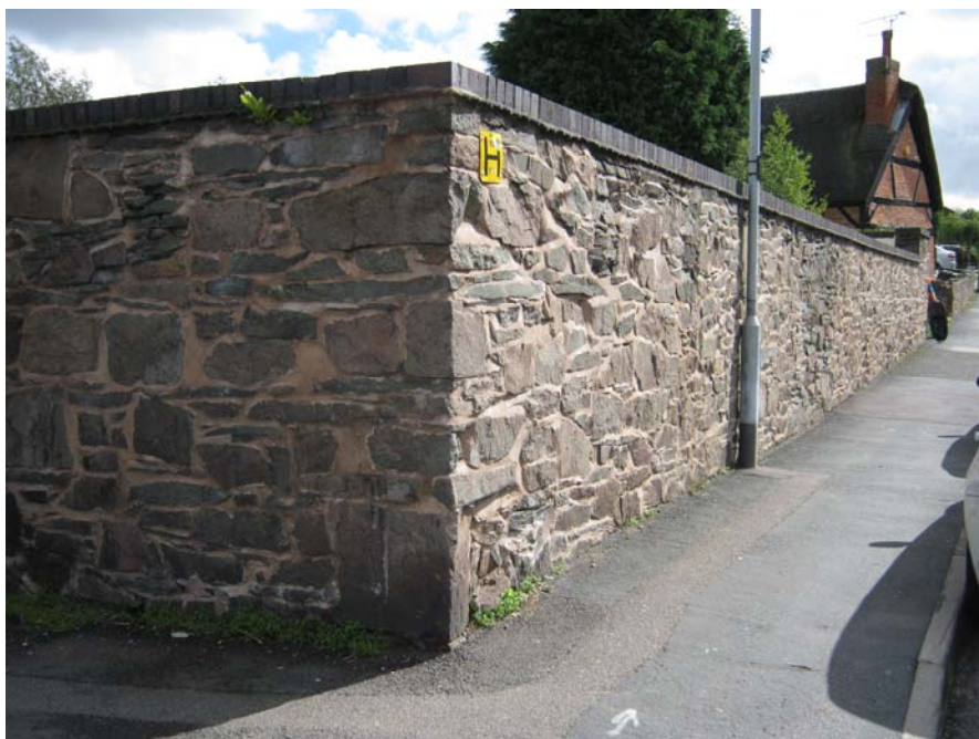
The attractive granite wall sited at the junction of Rookery Lane and Ratby Road helps to restrict views into the Stamford Arms pub car park.
