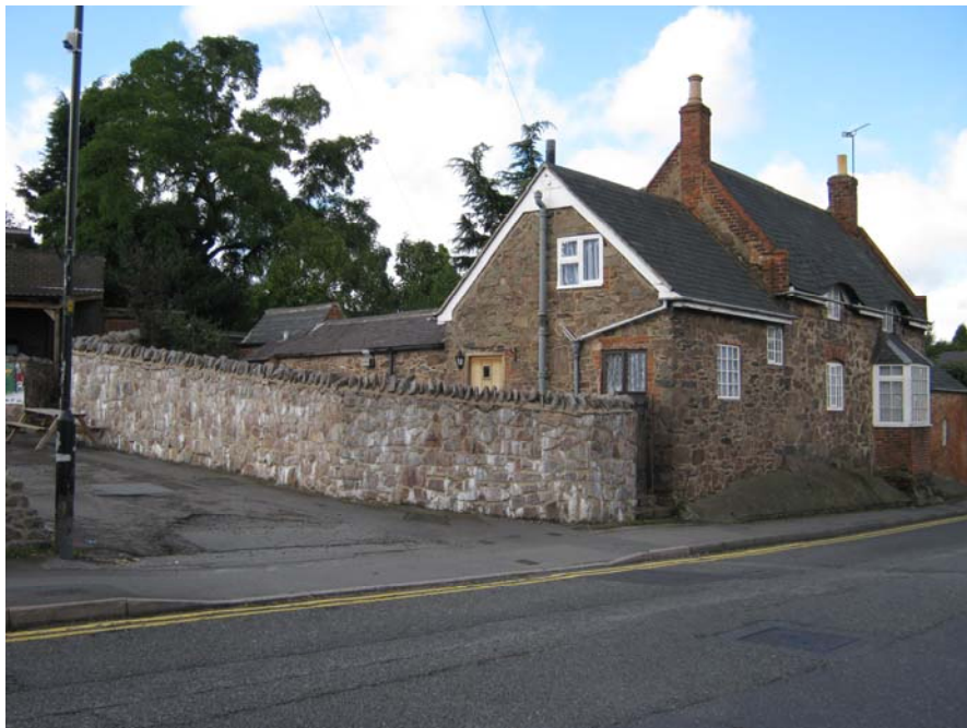
The Grade II listed C17 cottage, 12 Leicester Road, built in randomly coursed Mountsorrel granite with two eyebrow dormers, a front bay window and a slate roof.
