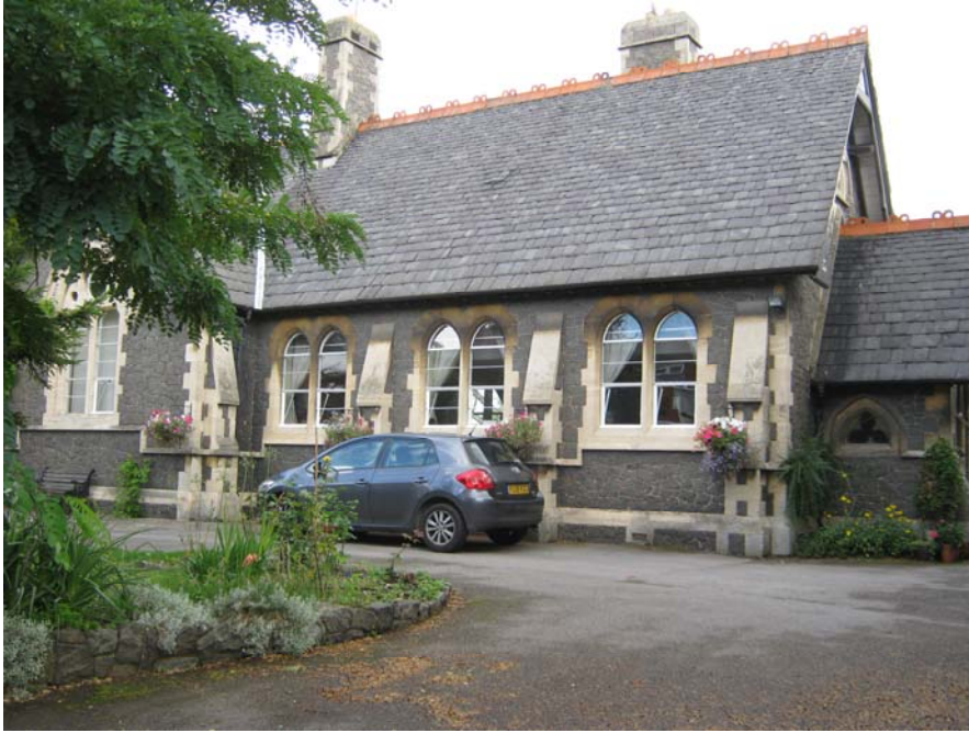
The former village school, 53 Leicester Road, is a Grade II listed building built in 1873. Built in random coursed rubble with ashlar dressings, slate roof and Gothic style cresting.
