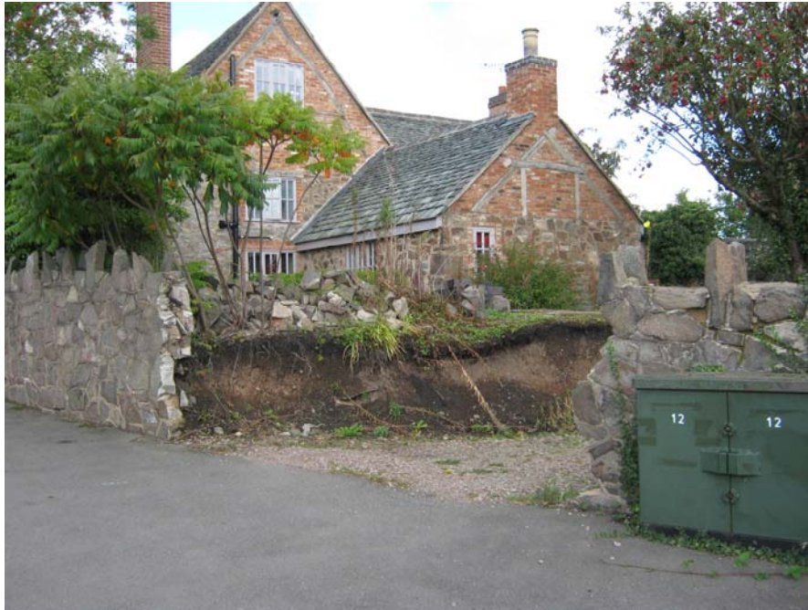
57 Leicester Road is an attractive timber framed cottage that has been modernised by having its roof raised and thatched roof replaced with slate. A new garage is to be constructed in the garden.
