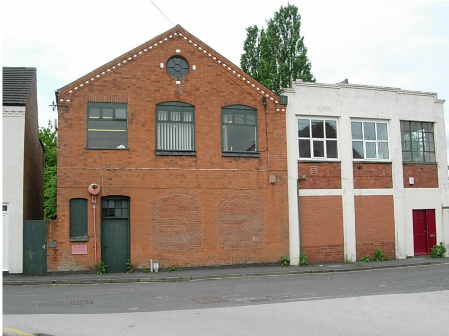
This fine former Victorian boot & shoe factory at the lower end of The Barracks was extended in 1930. Unfortunately the original windows have been replaced and two ground floor openings bricked up.
