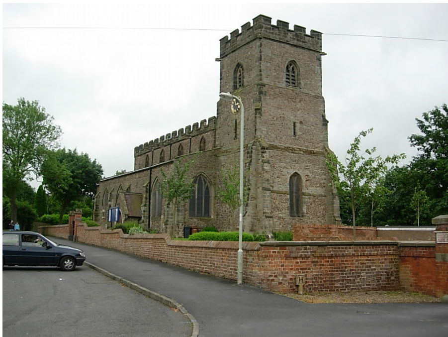
The Church of St Mary is a Grade 1 Listed Building, circa 1300-50 with late C15 clerestory built with random rubble and freestone dressings. The church is flanked by excellent traditional brick walls
