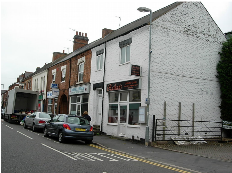
The style of rendering used on the gable of this property detracts from its appearance.
