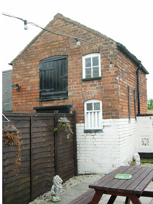
An alternative view of the same public house out buildings.
