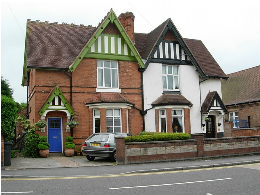
This fine house is very well maintained and has improved this part of the conservation area. The adjacent property has unfortunately lost some of its original features.
