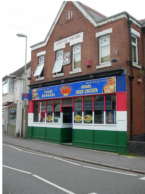
The over dominant signage, multi-coloured frontage and roller shutter on London House has a detrimental impact on its appearance.
