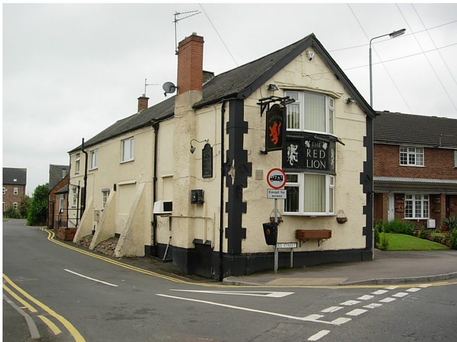
The Red Lion Pub, sited at the junction of High Street & Mill Street, is a striking rendered building that unfortunately has had its chimney stacks re-built.
