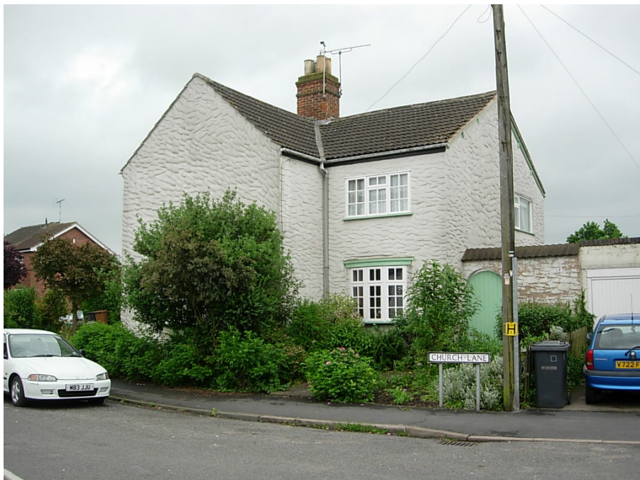
The property, 3 Church Lane, has lost most of its traditional character due to the modernisation of its windows and roof and inappropriate style of render.
