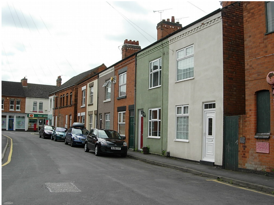
The unity of 1-11 The Barracks is lost by the multi-coloured rendering and re-constructed window openings. The properties still retain their original imposing chimneys and several stone window lintels.
