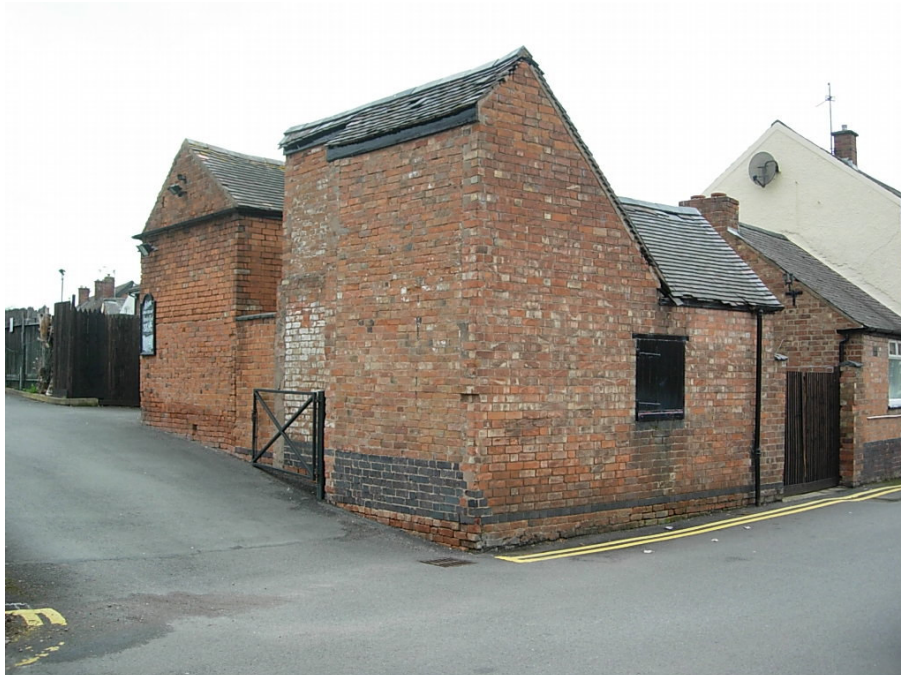
This group of small outbuildings at the rear of the Red Lion Inn adds significantly to the overall appearance of Barwell Lane.
